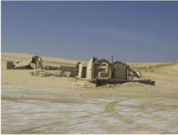
Fig. 15. Remains of the Rebro Haddada set (point C in Fig. 4), also used in the filming of Star Wars Episode 1. The roof collapsed under the weight of sand when the building was overrun circa 2005 and serves as an indication of what damage may be incurred by barchan passage over the Mos Espa site.
