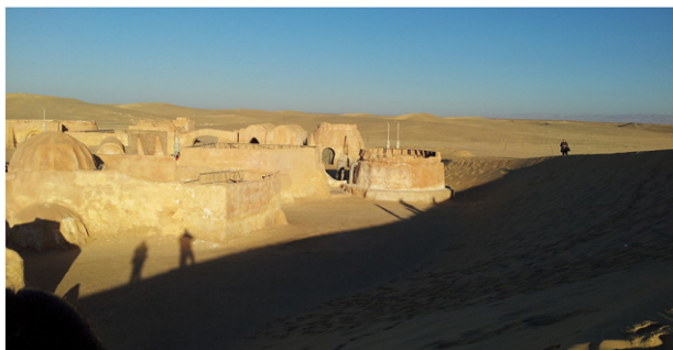
Fig. 18. A photo (courtesy of S. Slater) from the threat barchan crest looking northwest towards buildings A and B. This photo (acquired in December 2012) shows that the edge of the barchan is essentially in contact with building B (compare with images in Fig. 6). This photo demonstrates the utility of tourist photos in monitoring the site.
